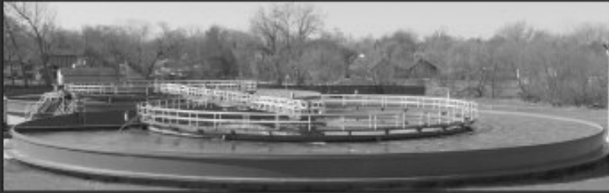
Wastewater Treatment Solutions
