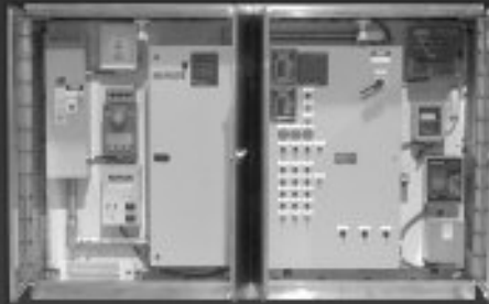
Pad Mounted Control Packages
